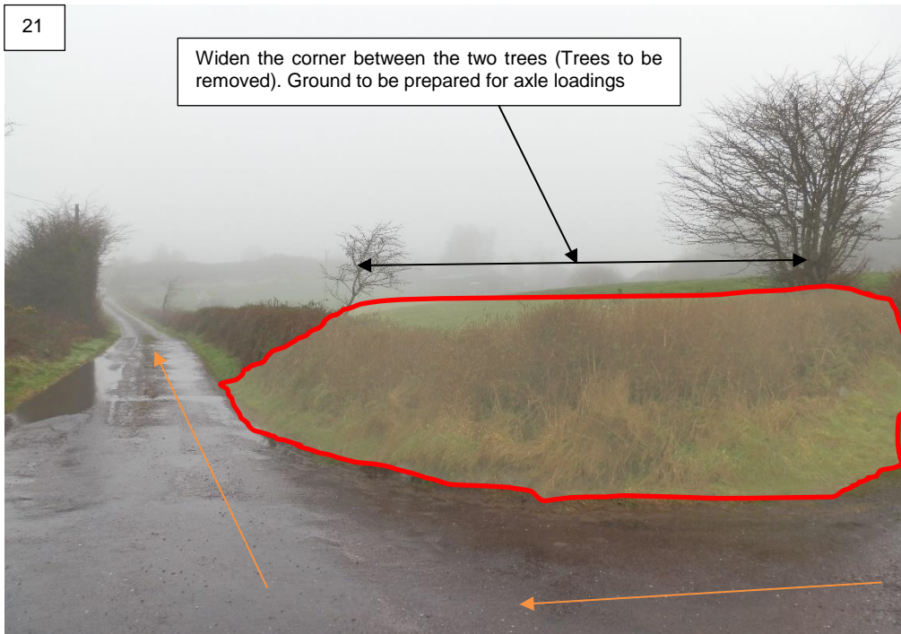
Route Marker 21– Right Hand Turn Prior to River Ilen. Widening works are required to the off side in order for the delivery vehicles to negotiate this junction.
