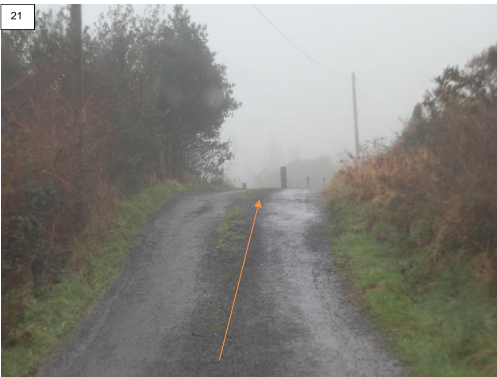
Route Marker 21 – Photo 5 the road surface is narrow and in poor condition Between 21 and 22, there are some undulations, which could cause a grounding Issue if trailers with low ground clearance are used..
