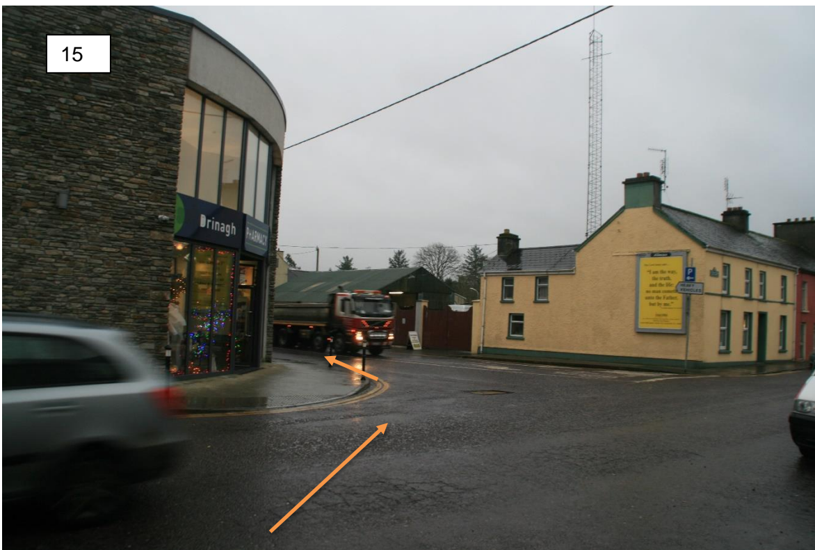
15 The left turn on to Sackville Street and the continuation on to Quarry Road is no issue.
