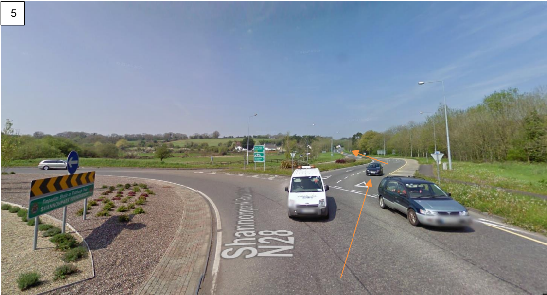
Route Marker 5 – Shannonpark Roundabout. The longer delivery vehicles such as the blades will require to travel contraflow around this roundabout. Shorter loads will be able to negotiate the roundabout in the usual manner.
