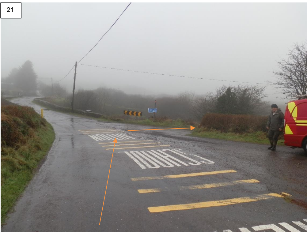
Route Marker 21 – Right Hand Turn Prior to River Ilen. Widening works are required to the off side in order for the delivery vehicles to negotiate this junction.
