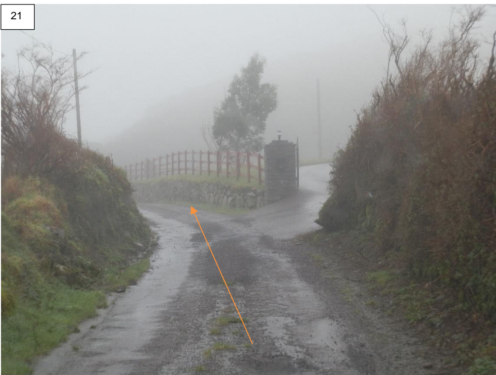
Route Marker 21 – Photo 3 There are number of points where the high banks will need to be Cut back/re shaped to allow the wide loads to pass
