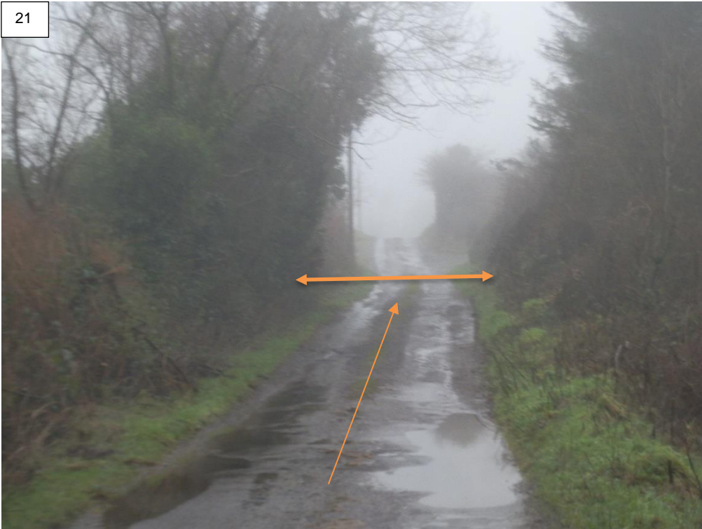
Route Marker 21 – Photo 2 Road side vegetation to be trimmed back
