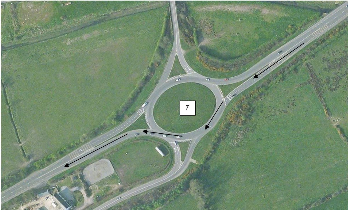
4.5.1 AERIAL VIEW OF ROUTE MARKER 7
