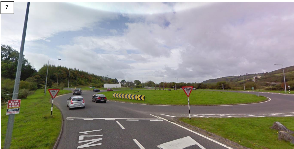
Route Marker 7 – N71 / R607 Roundabout. All vehicles will negotiate this roundabout without issue.
