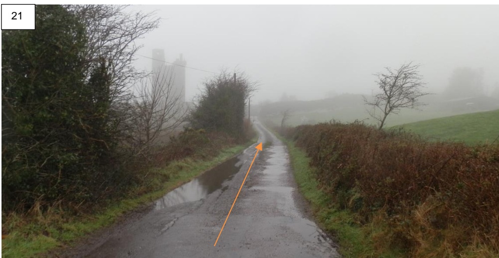
Route Marker 21 – Photo 1 Road and verges to be widened in accordance In accordance with Enercon specifications between markers 21 and 22
