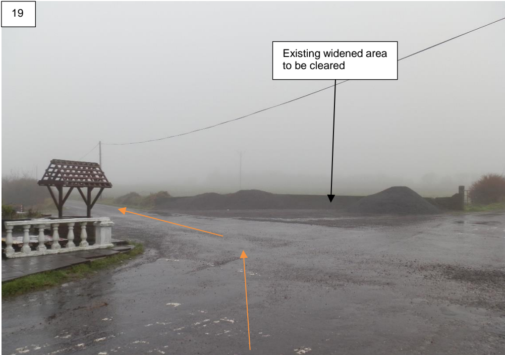
Route Marker 19 – Left Hand Turn onto Unnamed Rd. at Old Creamery. In order for the longer vehicles to negotiate this turn the existing widened area is required to be used. This area is currently being used to store road surfacing material.
